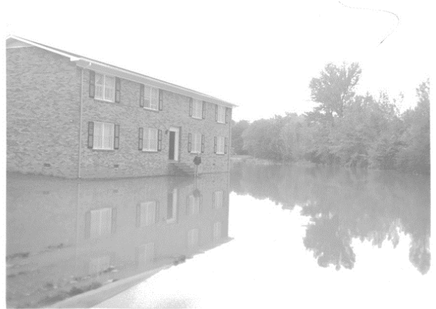
Flooding on Planation Road/ Meadow Drive after 5" rain 10-7-1970
